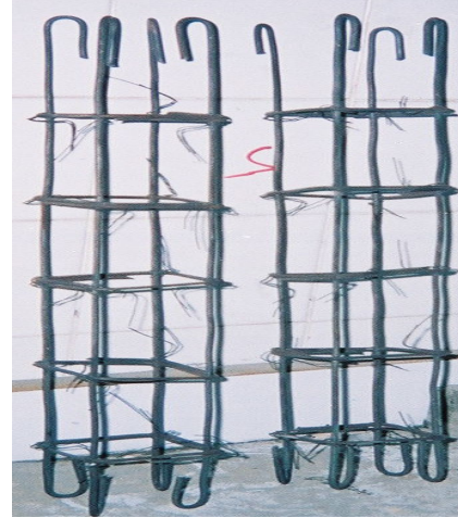
Figure 2 Reinforcement details of columns and ground beams
