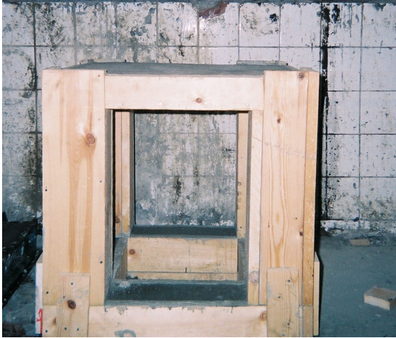
Figure 1 Model frame formwork
